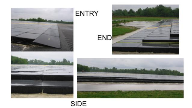
Figure 1.3. Adams Field EMAS Installation
