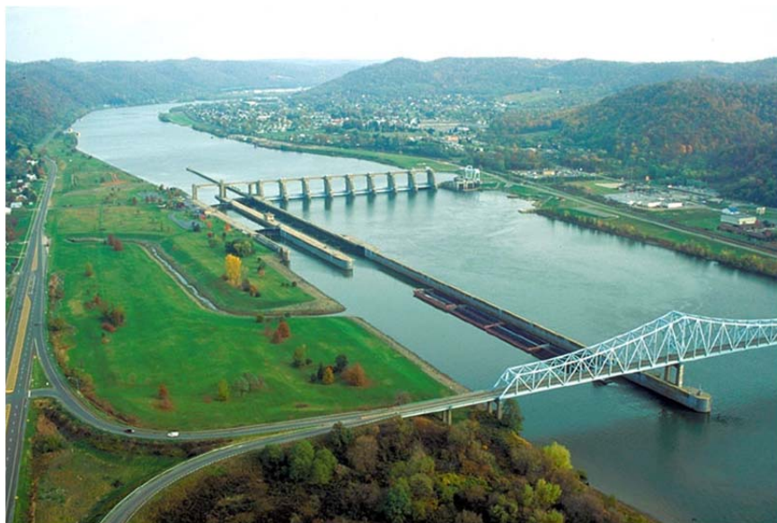
Figure 7: Hannibal Lock and Dam on the Ohio River has two navigation locks on the left and a hydropower plant on the right (Source: http://www.lrp.usace.army.mil/nav/hanni.htm )
