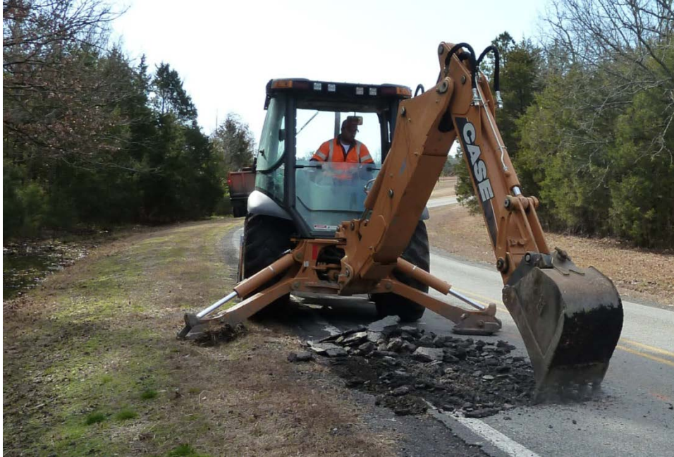
Figure 4 – Material removal from AR95
