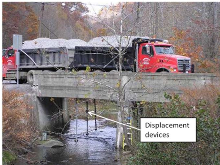
Figure 1.2: Static Bridge Testing Example
