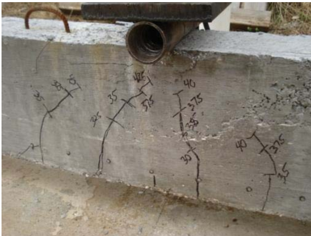
Figure 6.51: Cracking and failure of specimen NSL-4L
