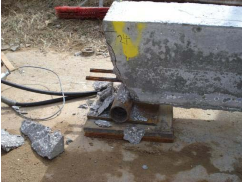
Figure 6.42: Spalling at support of specimen NSL-2D
