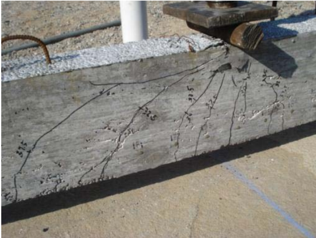
Figure 6.21: Cracking behavior and beginning of failure of specimen NSS-2D
