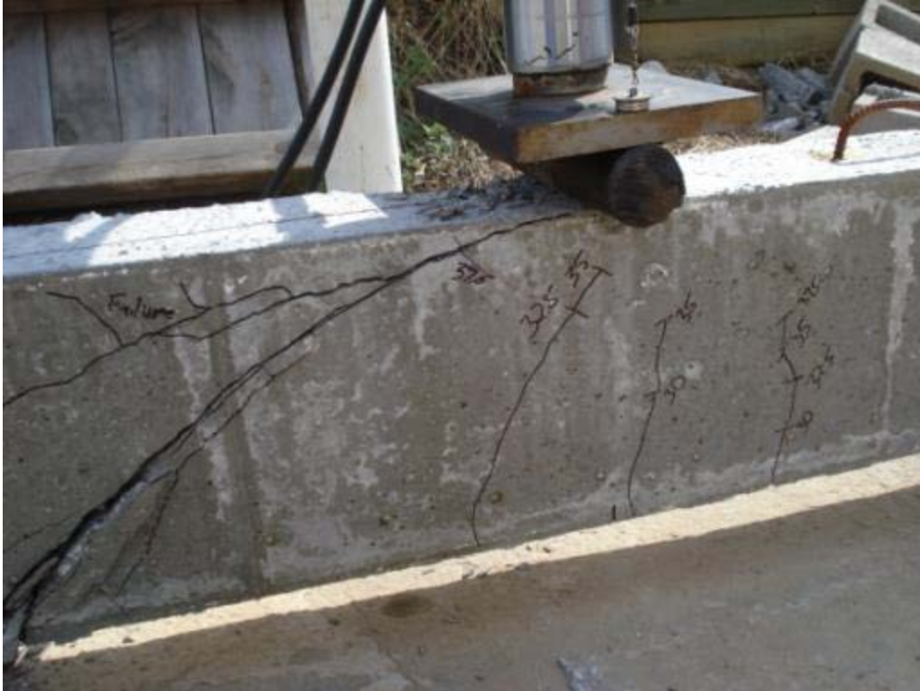
Figure 6.37: Shear cracking of specimen NSL-1D
