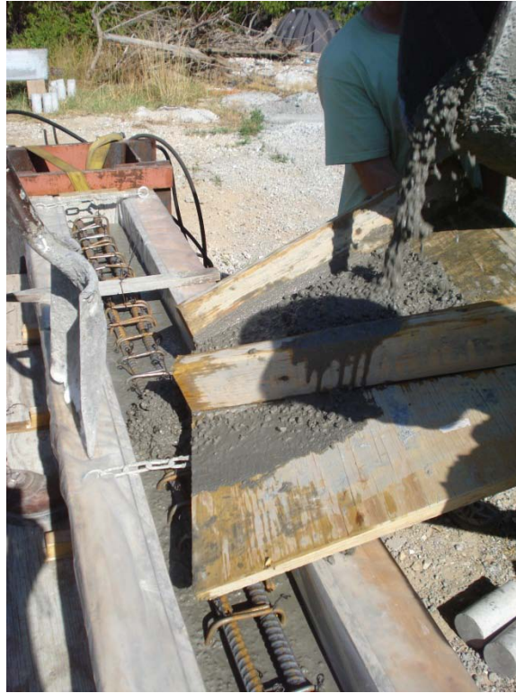
Figure 3.15: Concrete placement directly from the mixer
