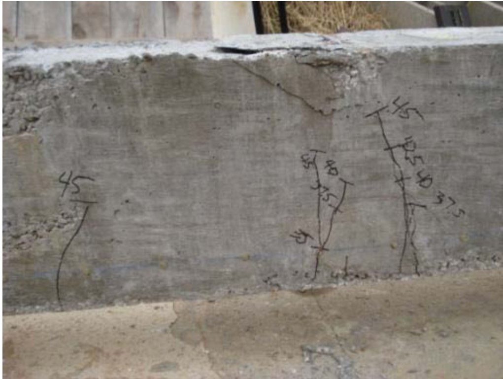
Figure 6.48: Cracking and failure of specimen NSL-3L
