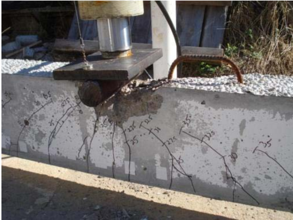
Figure 6.1: Cracking pattern of specimen NSC-1D
