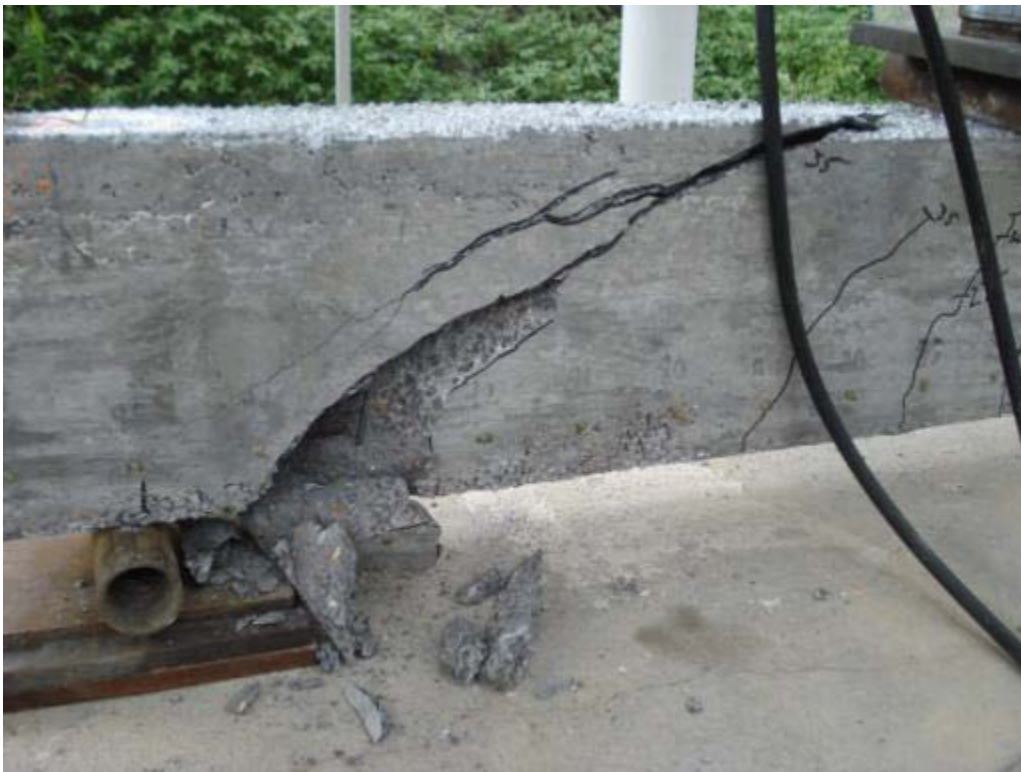
Figure 6.25: Shear failure of specimen NSS-3D
