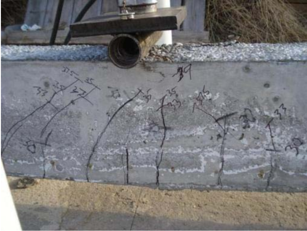
Figure 6.13: Cracking behavior of specimen NSC-4D
