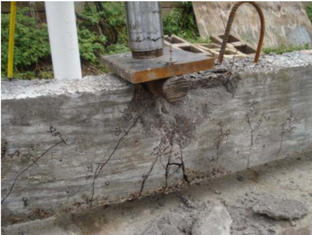
Figure 6.18: Cracking behavior and failure of specimen NSS-1D
