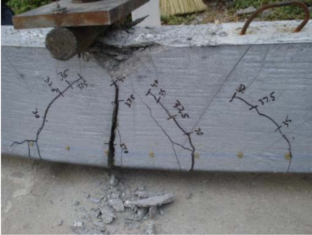
Figure 6.94: Cracking and failure of specimen HSL-3D
