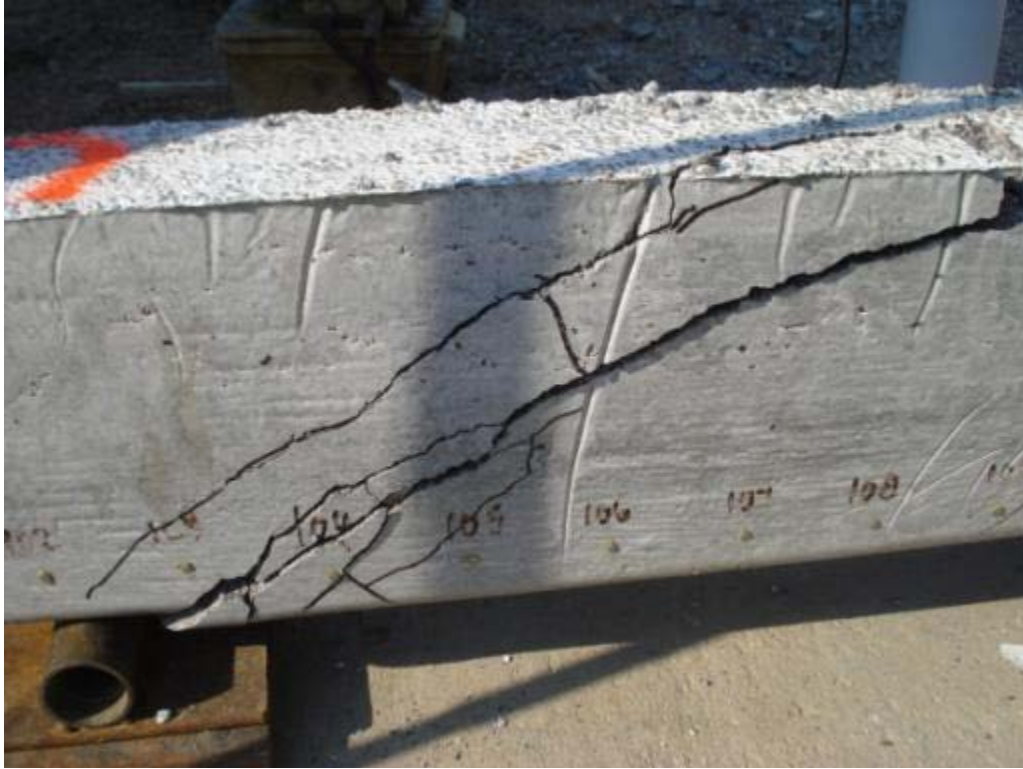
Figure 6.32: South side shear cracking of specimen NSS-4L
