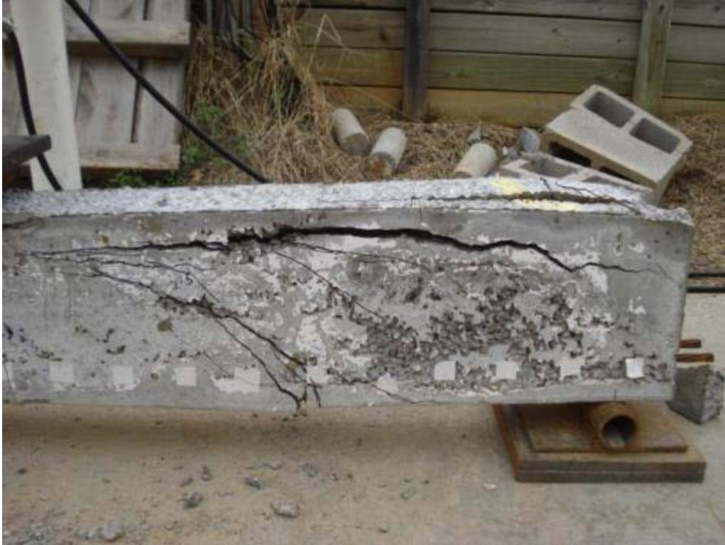
Figure 6.3: Shear cracking and poor consolidation of specimen NSC-1L
