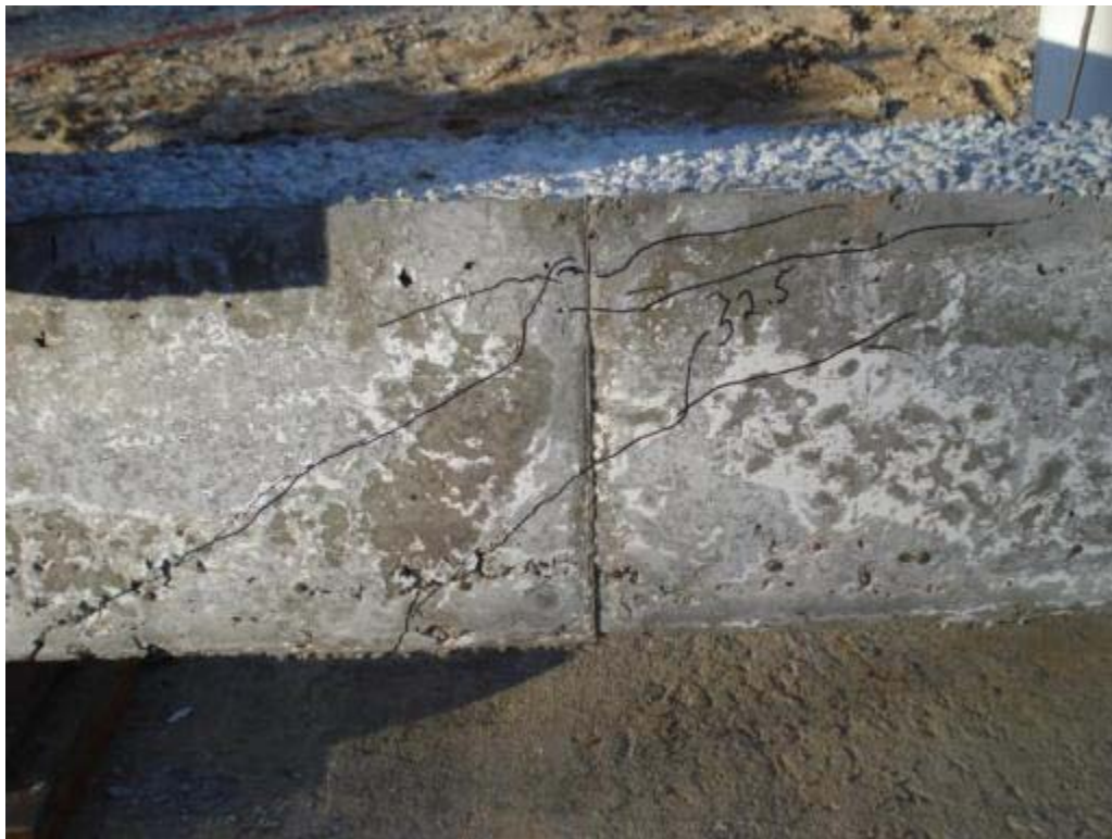
Figure 6.11: Shear cracking of specimen NSC-3L
