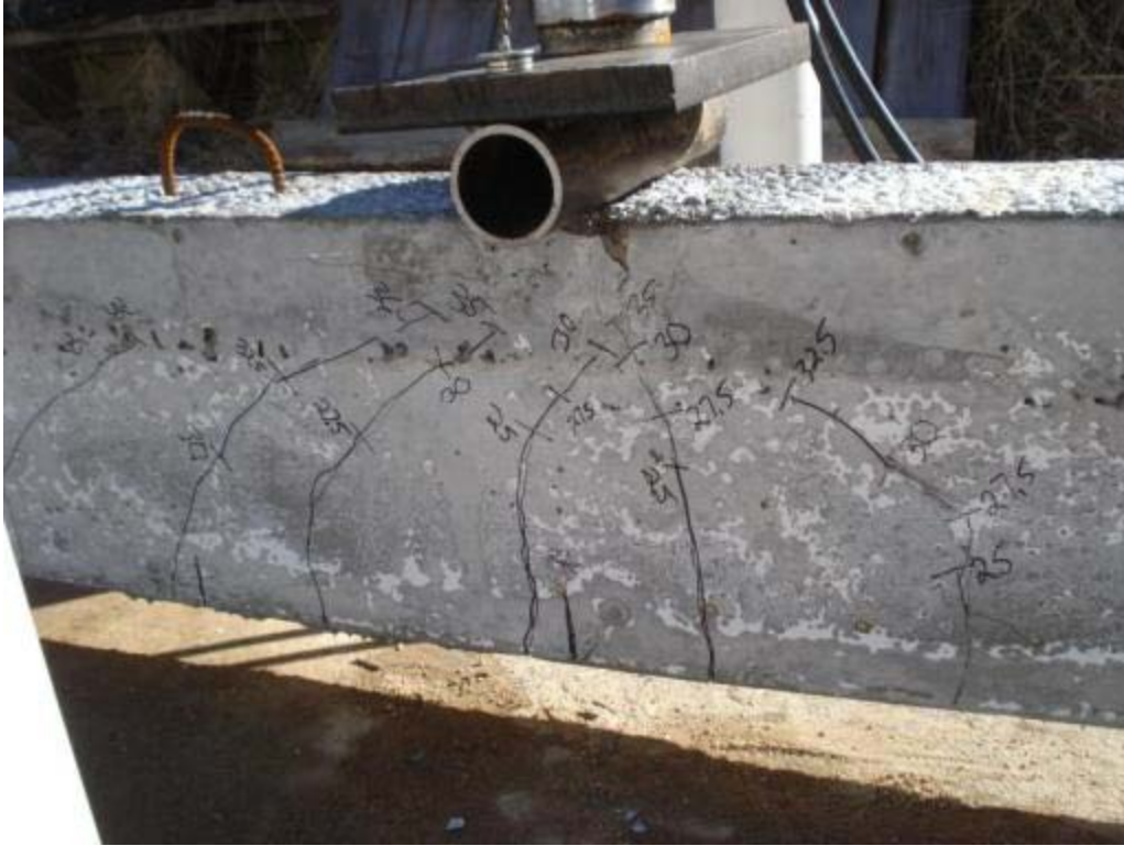
Figure 6.15: Cracking behavior of specimen NSC-4L
