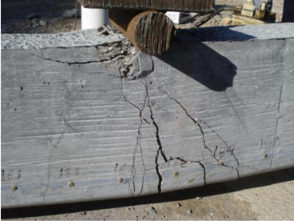
Figure 6.97: Cracking and failure of specimen HSL-4D
