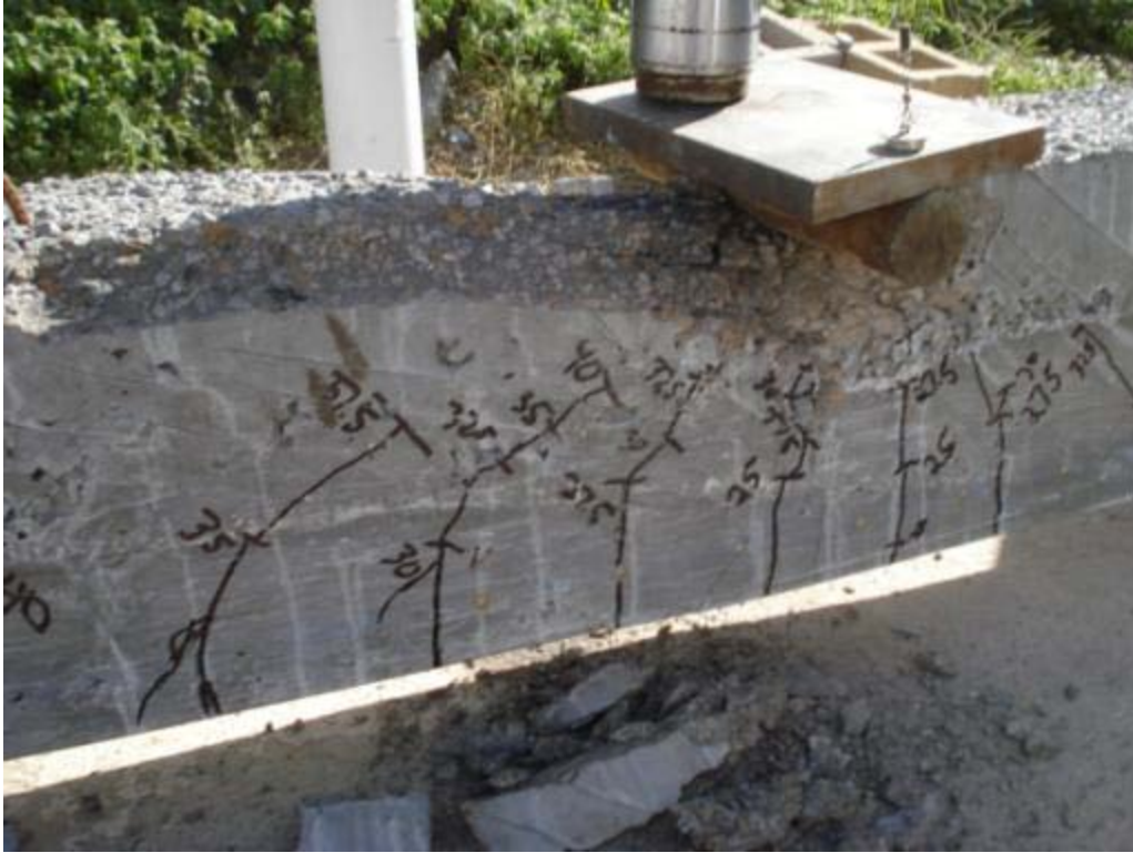
Figure 6.67: Cracking and failure of specimen HSC-4L
