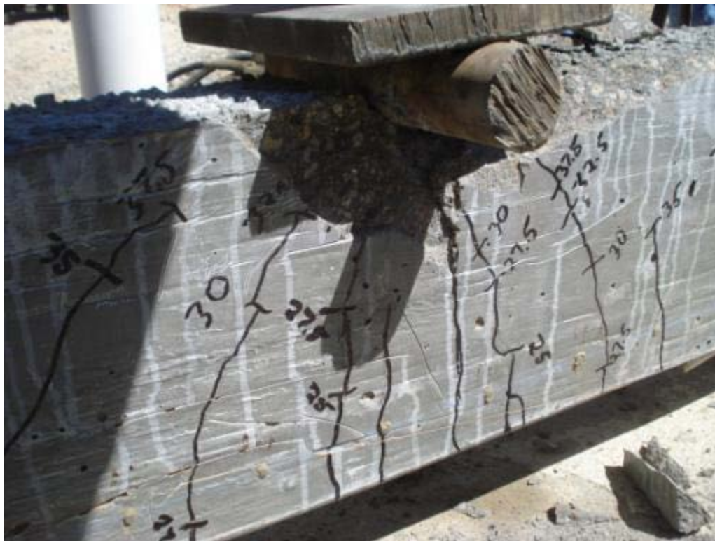
Figure 6.59: Cracking and failure of specimen HSC-2L
