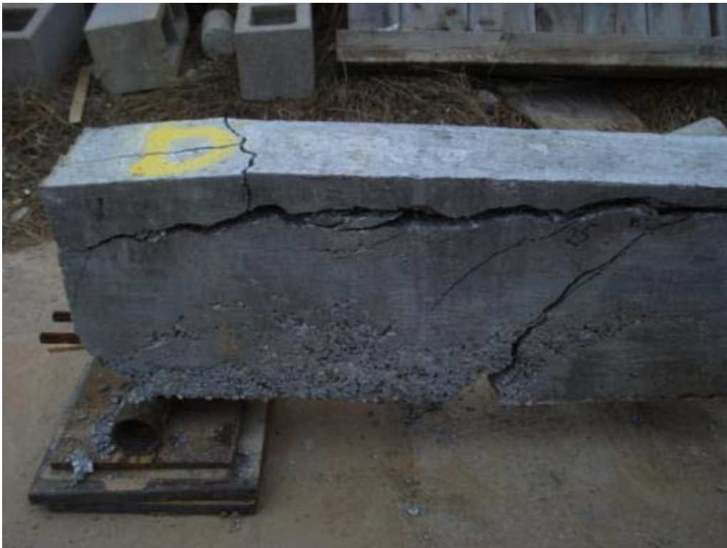
Figure 6.50: Shear cracking and failure of specimen NSL-4D
