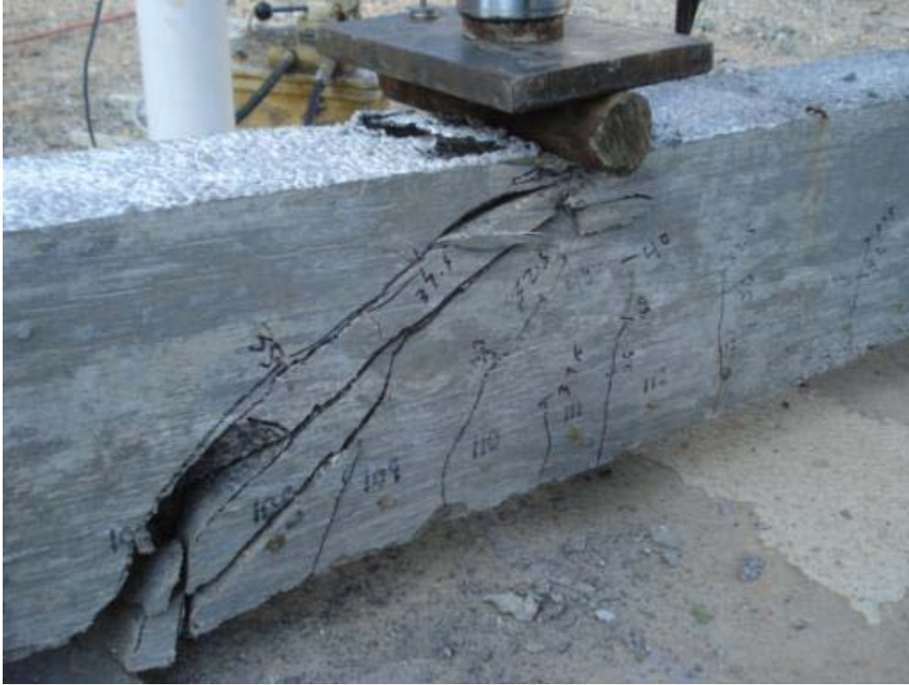
Figure 6.23: Shear failure of specimen NSS-2L
