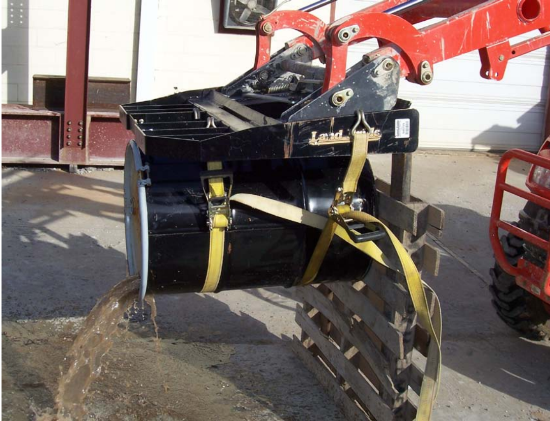
Figure 3.6: Aggregate preparation using steel drum and tractor loader
