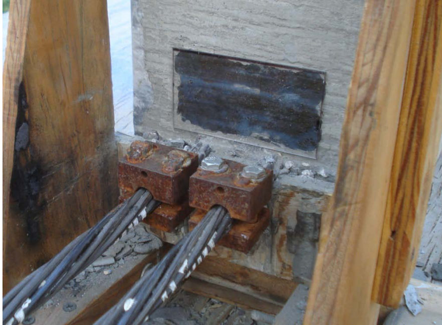
Figure 3.17: Placement of block clamps used to measure end slip
