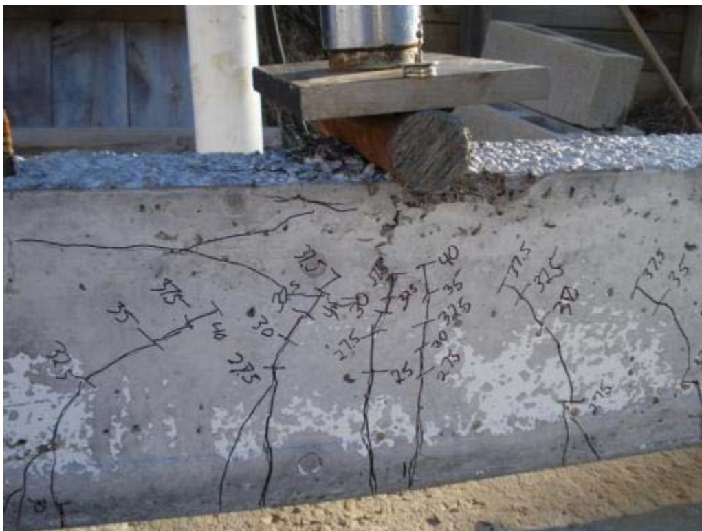
Figure 6.7: Cracking pattern of specimen NSC-2L
